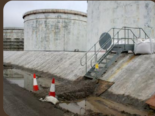
TANK FARM REMEDICATION
