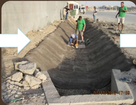
FORM A DITCH
